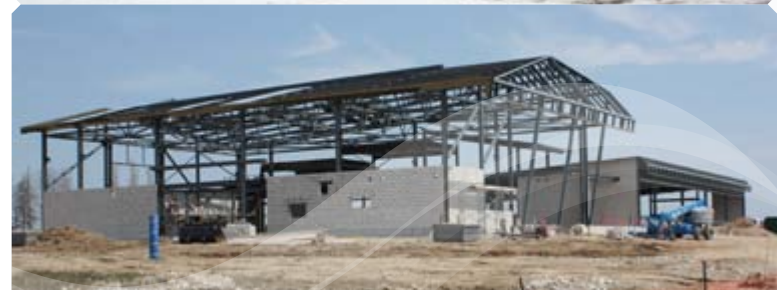
Construction of new facility from Nov. 23/08; Feb. 18/09; and April 24/09.
